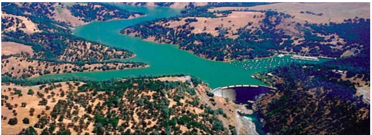
The reservoir above Englebright Dam on the Yuba River—a third filled up with sediment.
